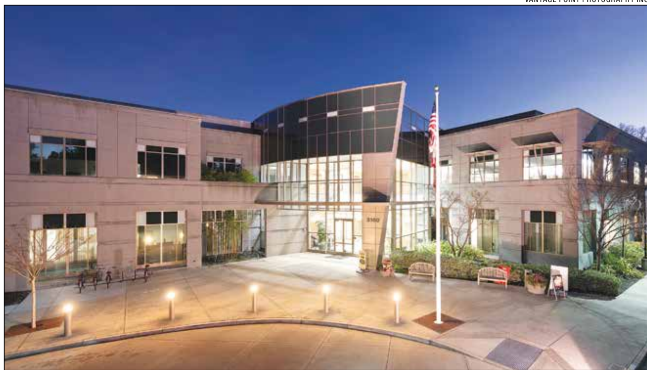
The 92,000-square-foot building at 3160 Porter Drive in Palo Alto will be developed into a life science incubator and small lab suites.
